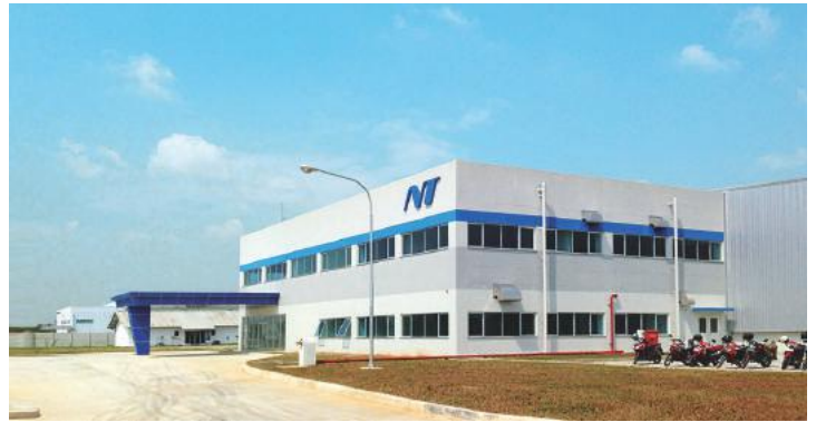
PT. NT INDONESIA (OFFICE/FACTORY)
